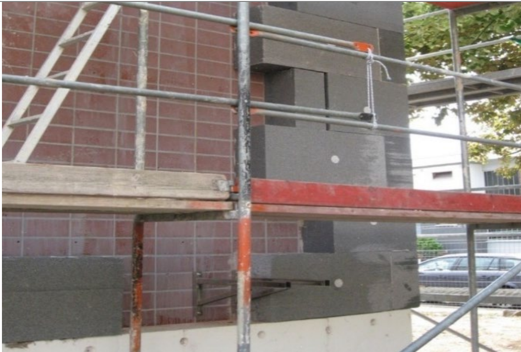
Figure 4 Insulating the walls of a building with polystyrene foam (Neopor) panels.
