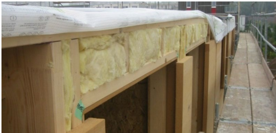
Figure 2 Insulation with mineral wool insulation materials.
