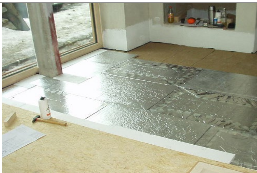
Figure 6 Insulating floors with vacuum insulation panels.
