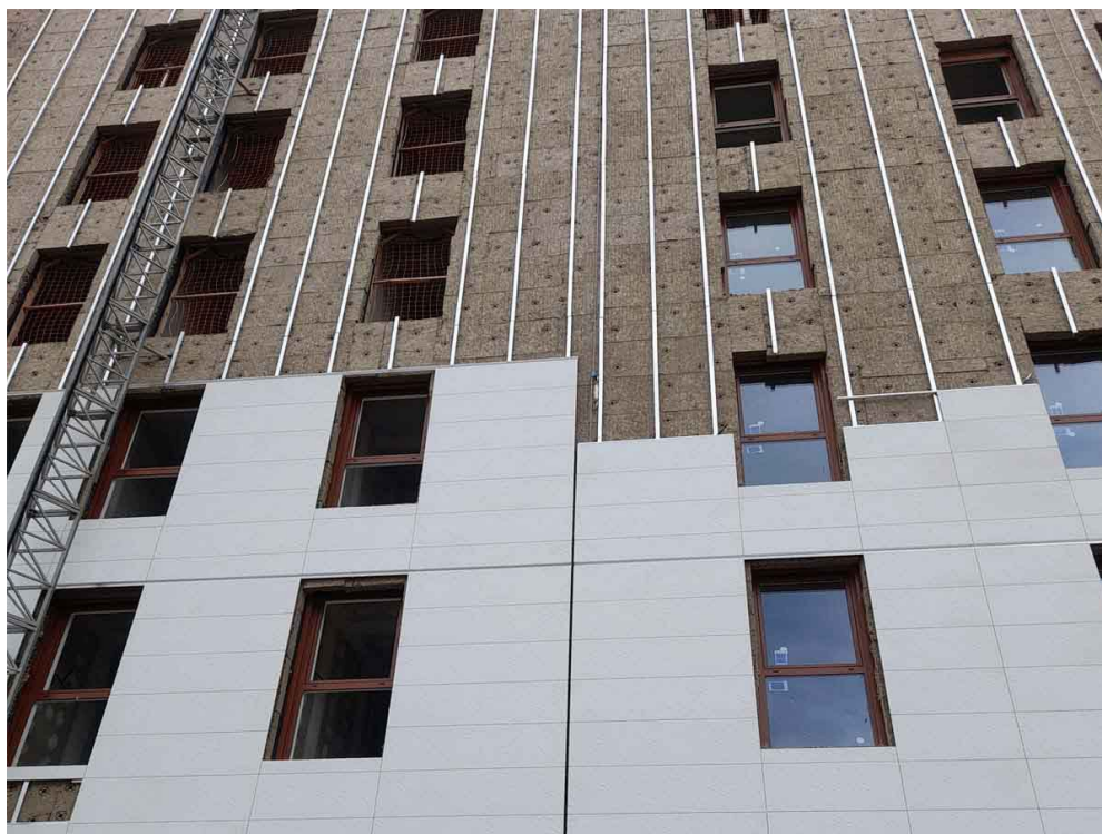
Figure 16: Energy rehabilitation of the façade. Ventilated façade
