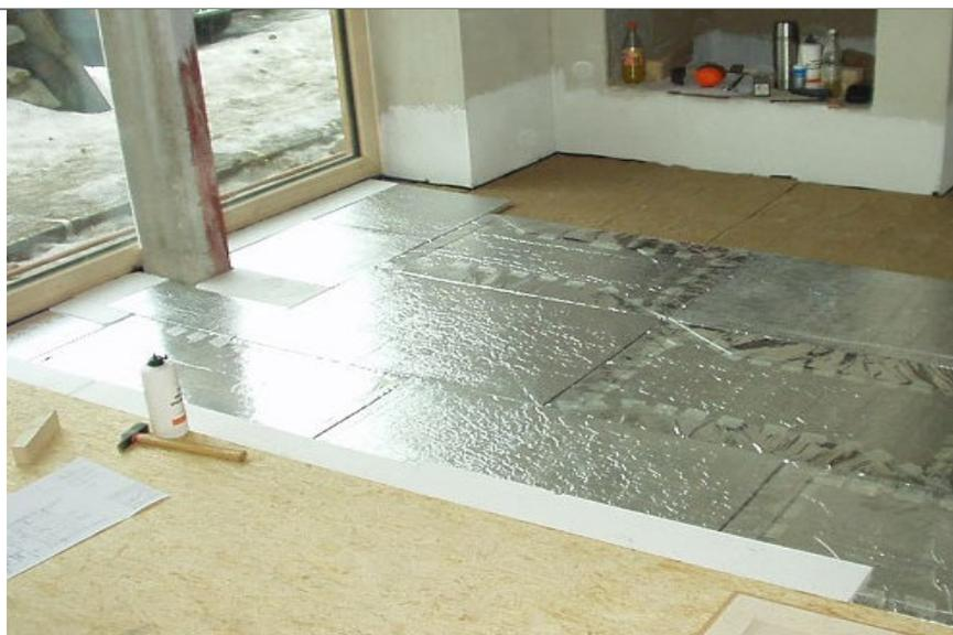
**Figure 6 Insulating floors with vacuum insulation panels.**
