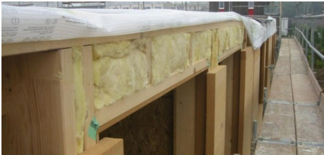
Figure 2 Insulation with mineral wool insulation materials.
